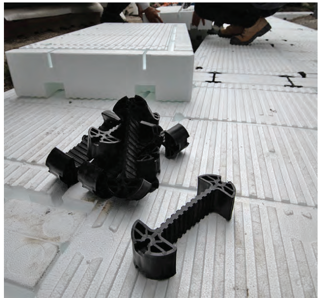
U-Core Connectors to lock units together
