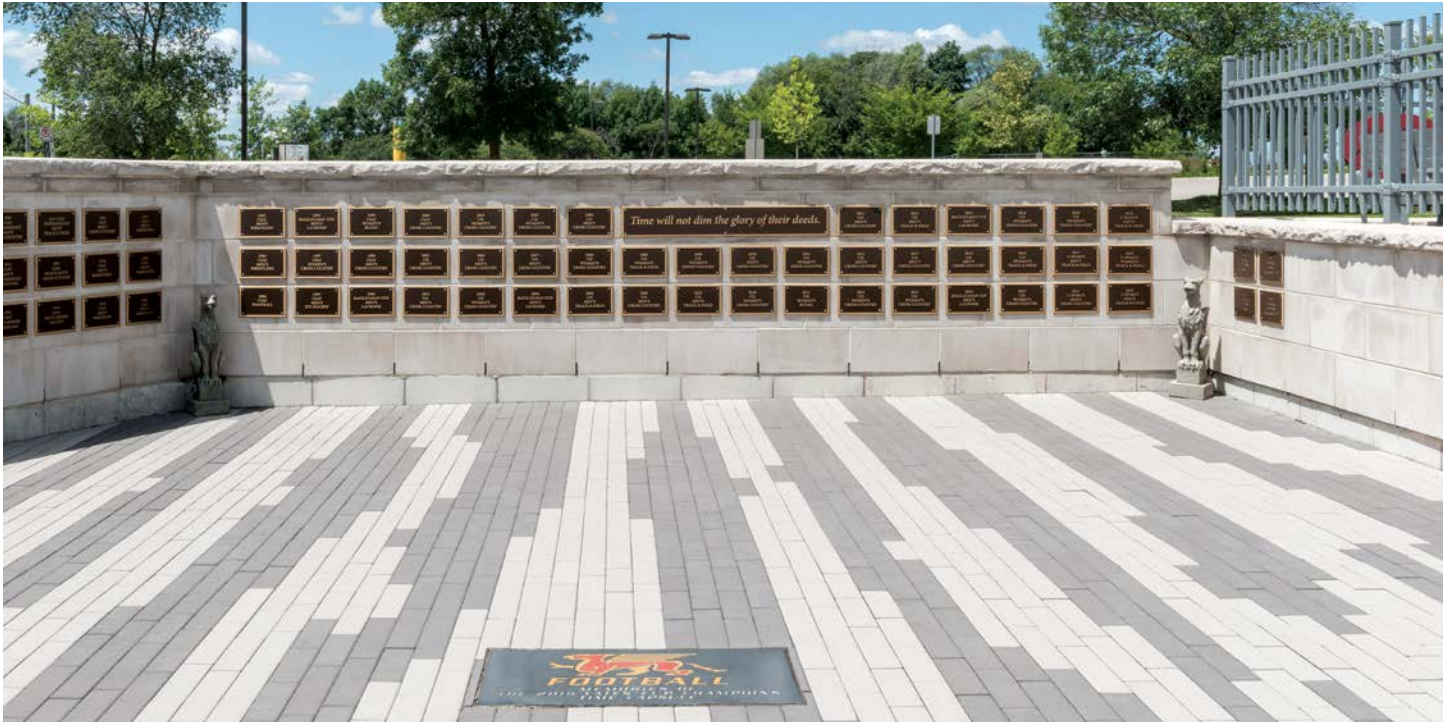
PROJECT: University of Guelph Stadium, Guelph, ON. DESIGN: Frontiers Design + Build. PRODUCT: 4 x 12" and 4 x 16" with Smooth Premier finish in Steel Grey and Opal.
