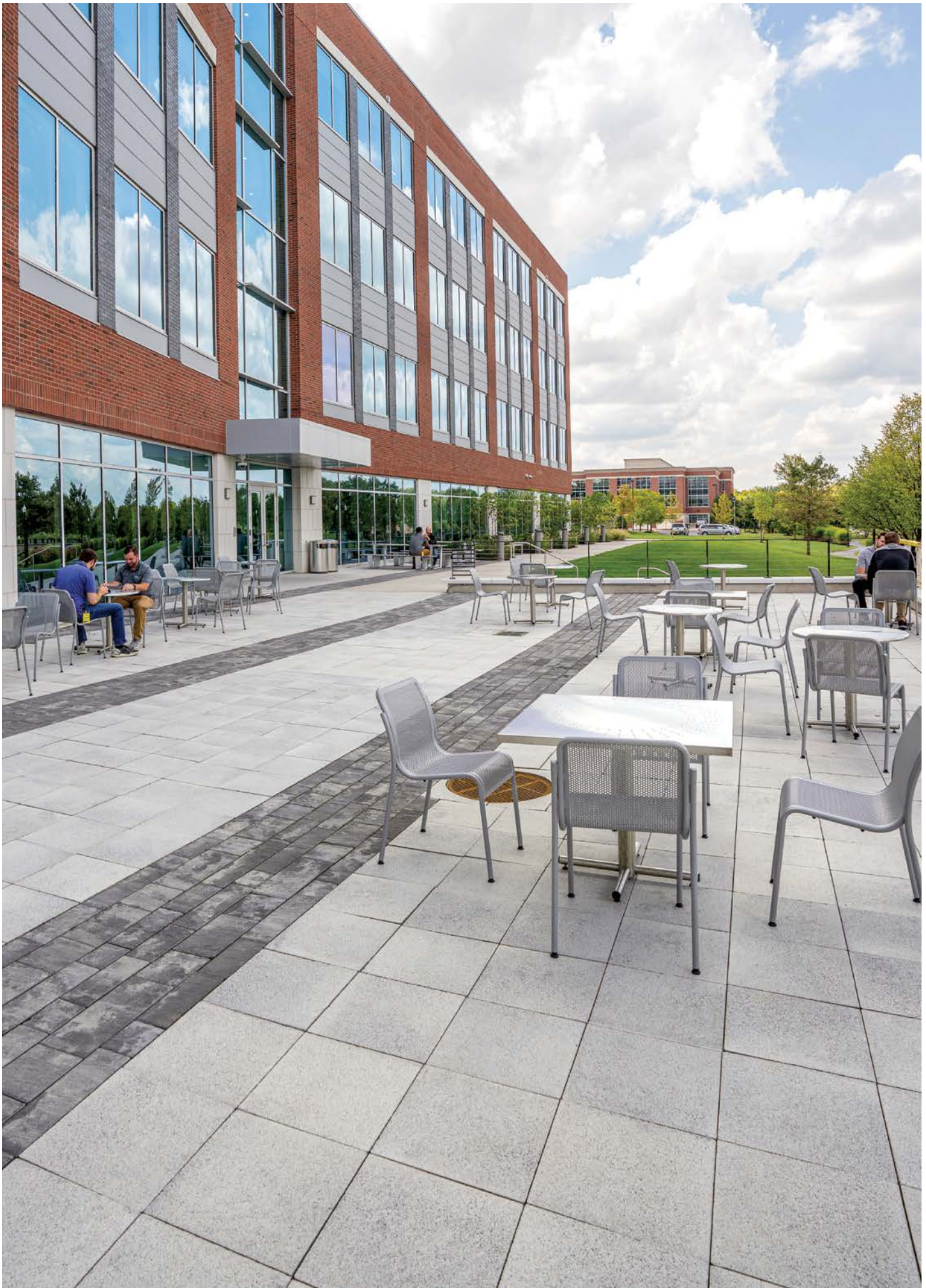
PROJECT: Private Company Headquarters, Westerville, OH. DESIGN: Edge Landscape Architecture. PRODUCT: 16 x 16" with Umbriano® finish in Winter Marvel and Artline™ with Il Campo® finish in Granite Fusion.
