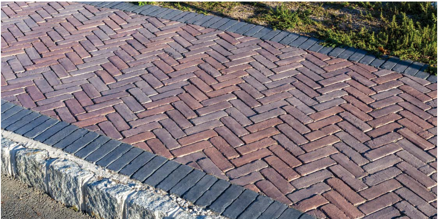
PROJECT: Allendale Streetscape, Allendale, NJ. DESIGN: Neglia - Engineering Associates. PRODUCT: Copthorne® in Burgundy Red, Burnt Clay, Old Oak, and Basalt.
