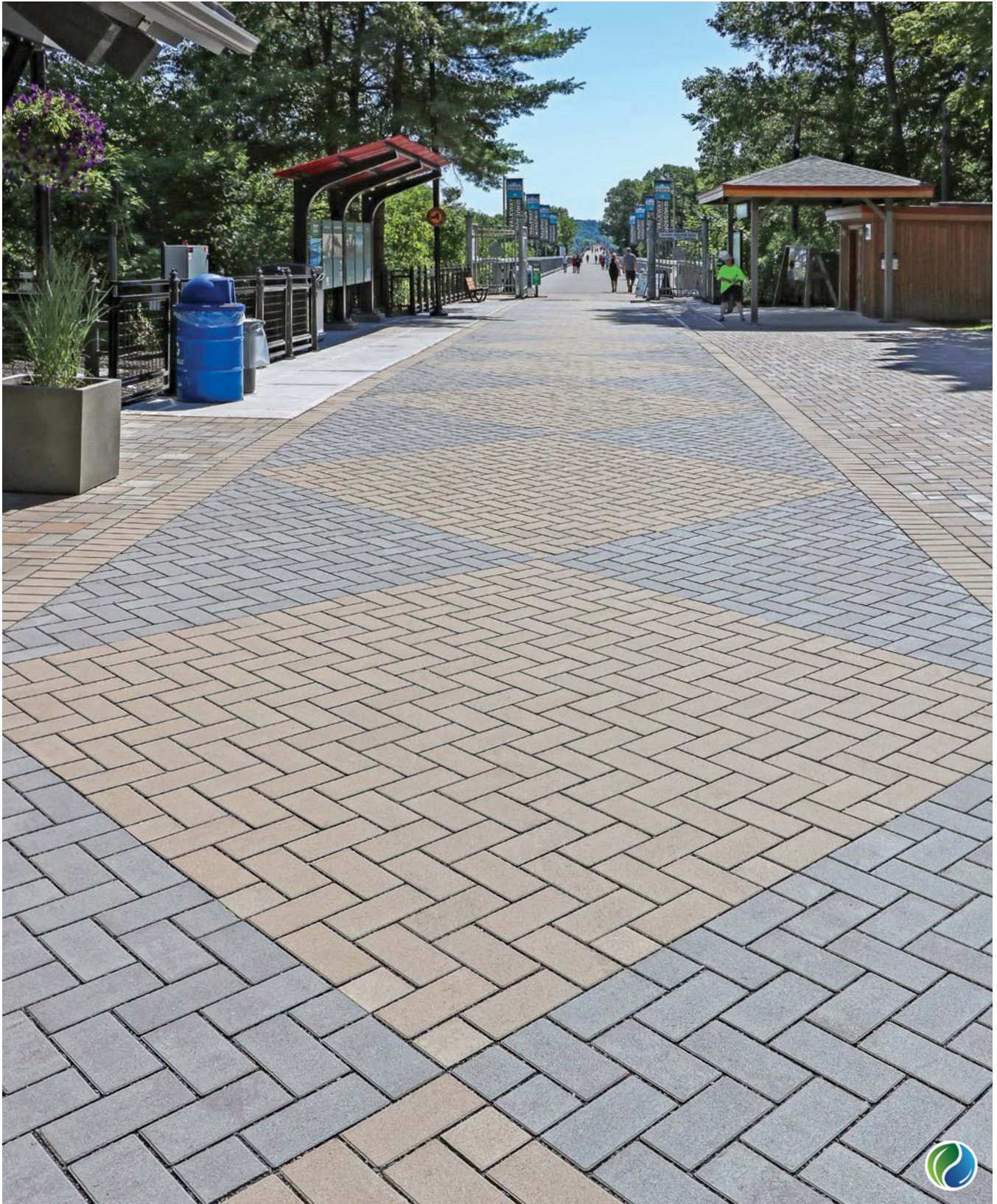
PROJECT: Walkway Over The Hudson, Poughkeepsie, NY. DESIGN: Saratoga Associates Landscape Architects. PRODUCT: 5 x 10" Permeable with Smooth Premier finish in New York Blend and Sandstone.
