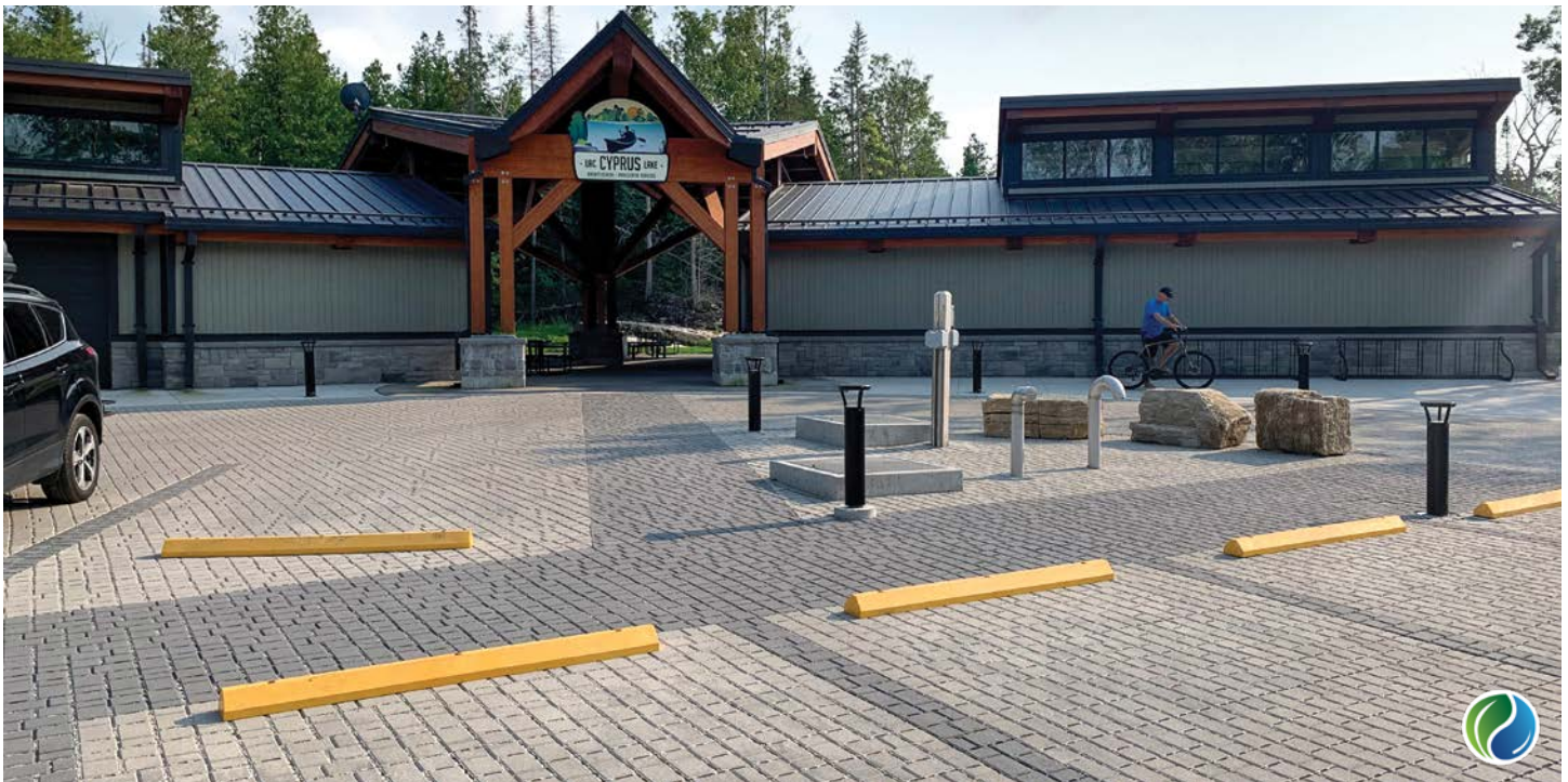
PROJECT: Bruce Peninsula National Park - Cyprus Lake the Hub, Tobermory, ON. DESIGN: Aecom Kitchener. PRODUCT: Eco-Optiloc™ in Natural and Charcoal.
