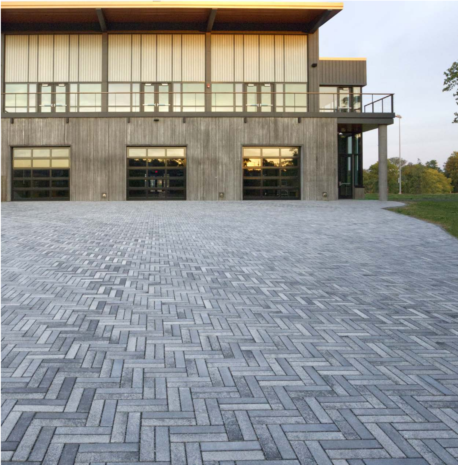
PROJECT: Bergen County Rowing Center, North Arlington, NJ. DESIGN: Clarke Caton Hintz. PRODUCT: 3 x 12" Permeable with Umbriano™ finish in French Grey and Winter Marvel.
