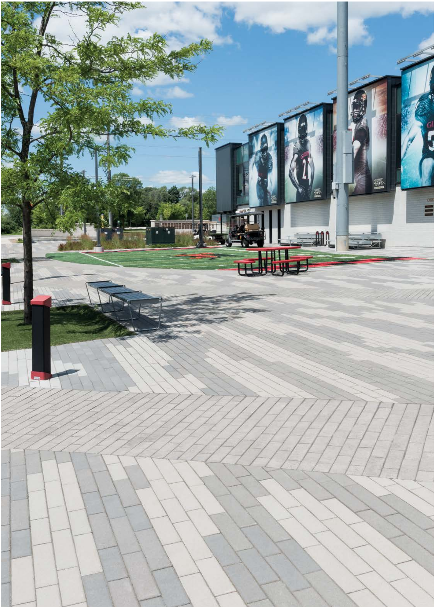
PROJECT: University of Guelph Stadium, Guelph, ON. DESIGN: Frontiers Design + Build. PRODUCT: 4 x 12" and 4 x 16" with Smooth Premier finish in Steel Grey and Opal and Il Campo® finish in Granite Blend.
