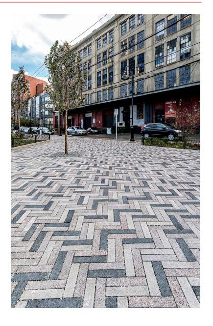
"The shapes, colors, and finishes of Unilock permeable pavers provided many design options for the park plaza and paths and assisted with stormwater management"
